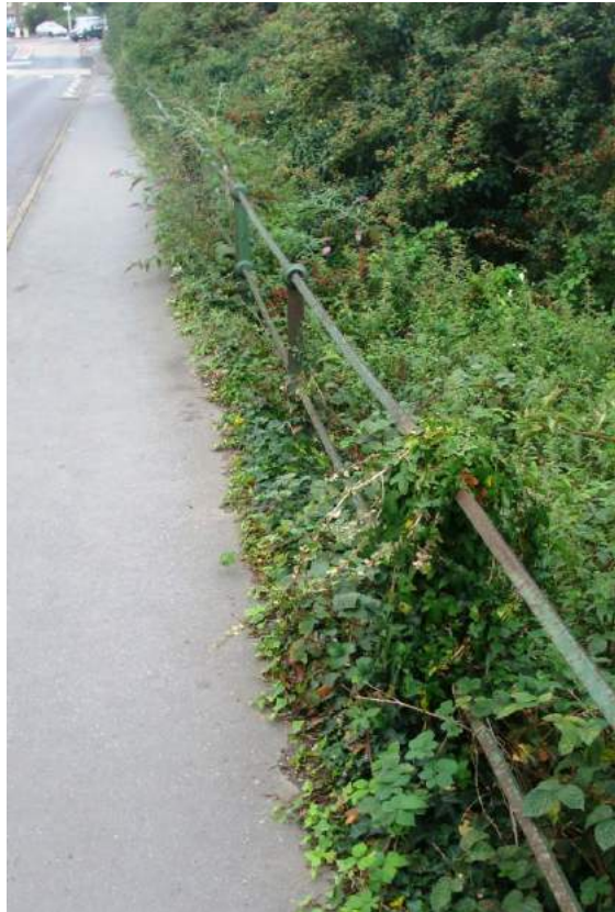
Picture 51. Low railings less than 1m in height and thus unprotected from demolition within the Conservation Area. Potential candidates for formal protection by Article 4 Direction. Need to remove vegetation repair and repaint. In first instance need to discuss issue with Thames Water if indeed they are the owners.
