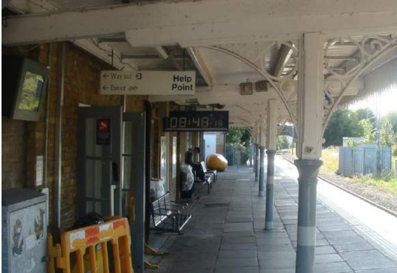
Picture 50. 19th century station part of the industrial heritage of the town. Canopy and cast iron supports are typical.
